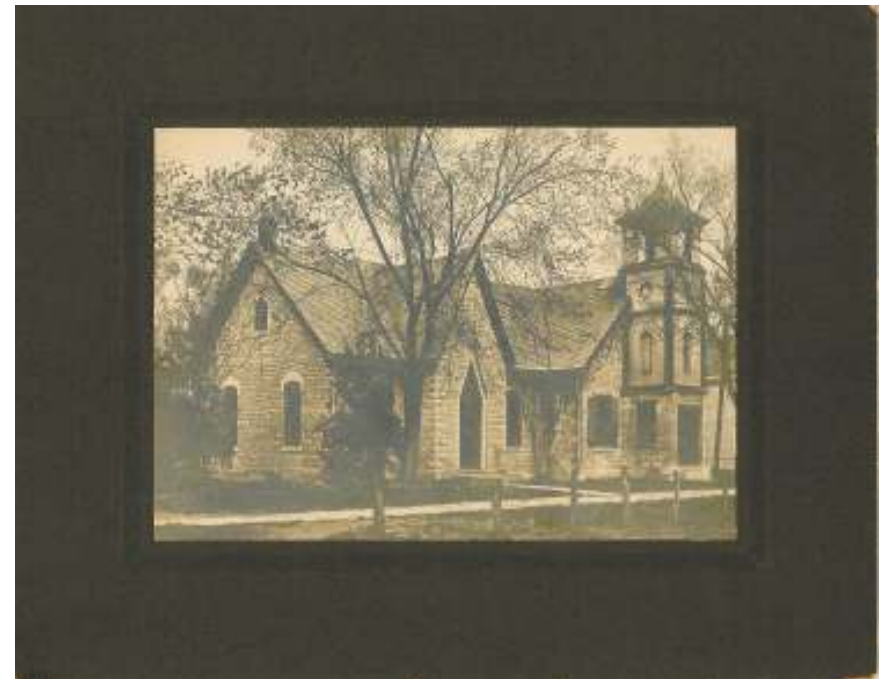
Constructed in 1858-1859, Pioneer Hall (on the right) is seen with its first addition (now incorporated into Blachly Hall) in this photo from the 1870's,
